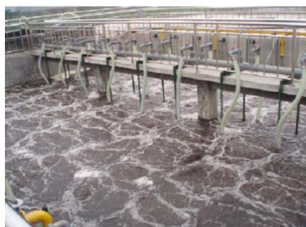
Fig. 2: Submerged Membrane Bioreactor
