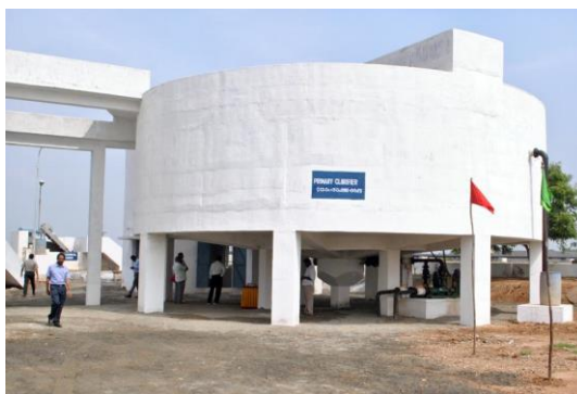
Fig.4 : Elevated Primary Clarifier
