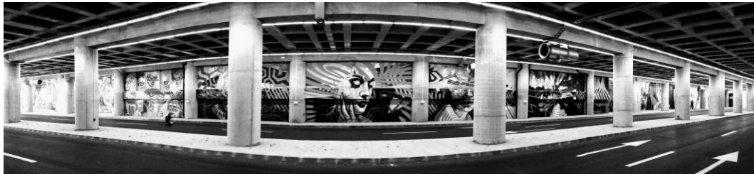
Fig. 5: Circular apparent concrete collumns of the Undertown Street Art Gallery
