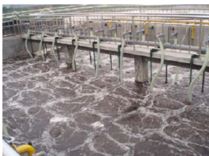
Fig. 2: Submerged Membrane Bioreactor
