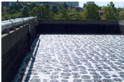
Fig.6 - CETP in Istanbul, Turkey with Sea discharge for TDS management
